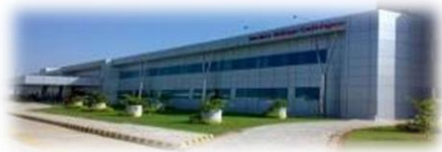
MV/ LV Equipment Vadodara (VDR)
